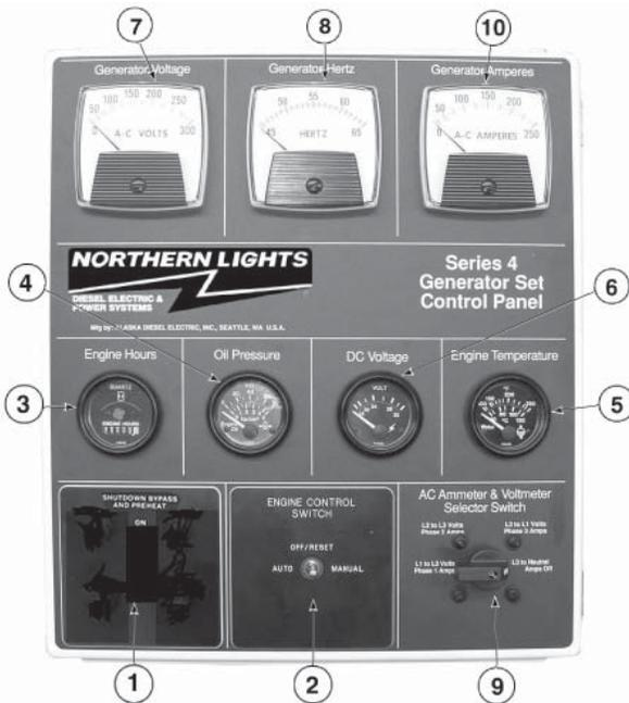
Figure 4-C: Series 4 Generator Control Panel
