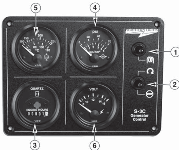
Figure 6-a: Series 3 Generator Control Panel
